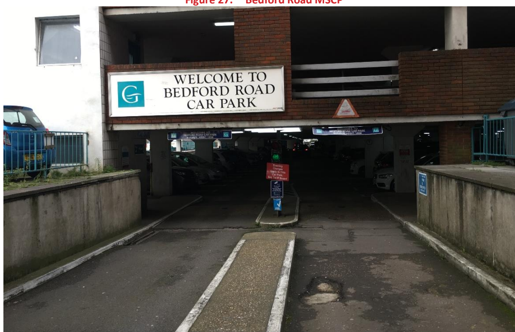
Figure 27. Bedford Road MSCP
