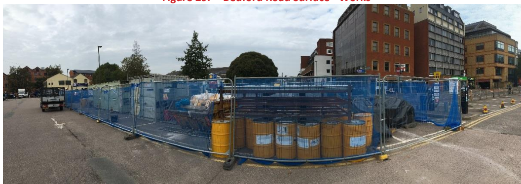
Figure 29. Bedford Road Surface - Works
